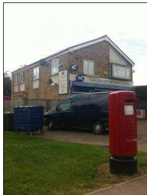
Caldecote Stores. A small convenience store in Upper Caldecote
