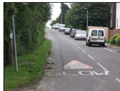
Lack of footpath on approach to Stondon Lower School
