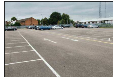
Under utilised station car park, Biggleswade
